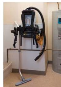
A sturdy steel wall bracket is mounted to the wall with three screws. The Vac Station attaches to the bracket and allows for 20" of travel. Crevice tools and floor tools slide into holes behind the vacuum. Extension cords hang from the side.
